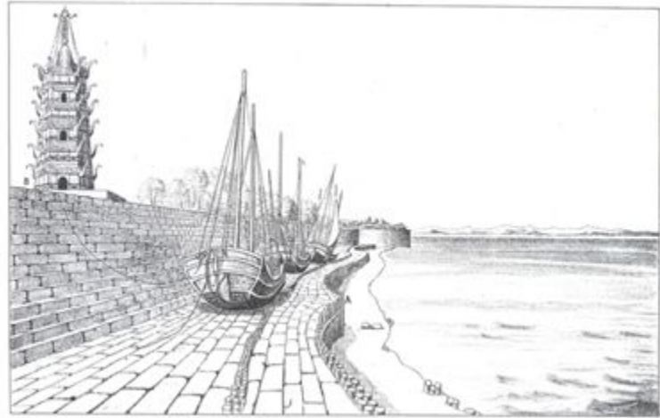
BORE SHELTER FOR JUNKS, AT BHOTA PAGODA HAINING. The point A is 7 feet, & B is 218 feet, above low Water Level.
